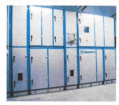
DesiCool<sup>TM</sup> is a complete air-conditioning system based on desiccant cooling. Although it uses no compressors, it has a capacity similar to conventional CFC-based systems. It is possible to cool ambient air at a temperature of 30 °C down to 15 °C. For the cooling process to function properly during the summer months, additional heat is needed. The more heat added, the coolerit gets! Excess heat can be made good use of.
