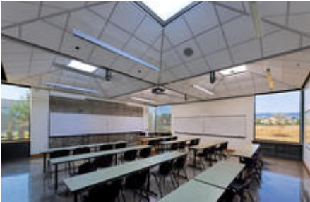
The daylighting strategy combines common skylights and acoustical ceiling tiles in a unique sloped ceiling system. - Photo Credit: Stephen Miller
