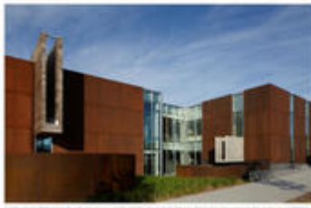
Stormwater Resue and Detention - Photo Credit: Kate Joyce Studios with diagram by Ross Barney Architects
