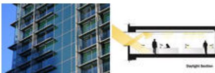
Because of the importance daylighting plays in human health and comfort, the project optimized daylighting in the perimeter zone utilizing a task/ambient approach to lighting. - Photo Credit: SERA
