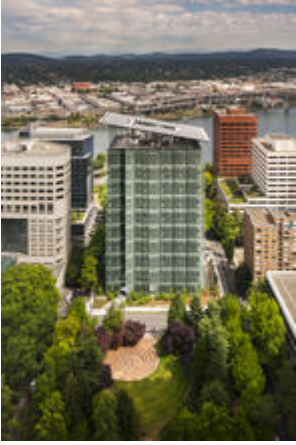
View from neighboring building, looking east - Photo Credit: Nic Lehoux
