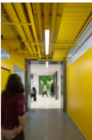
MEP and Other Systems Are Intentionally Left Exposed - Photo Credit: Photo © James Ewing
