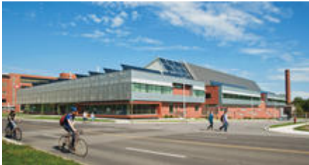
south-West corner along Longwood Road - Photo Credit: Elizabeth Gyde
