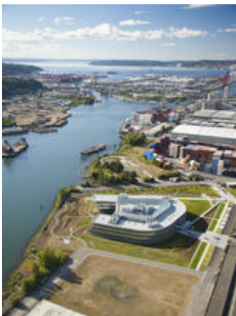
Aerial facing north - Photo
