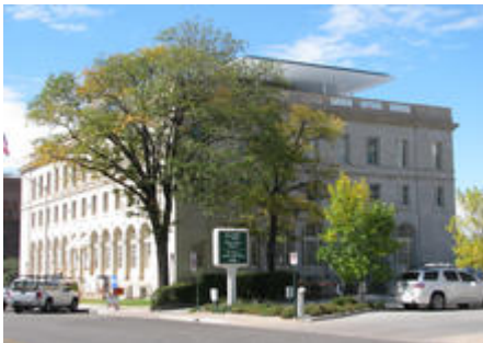
Southeast corner of building
