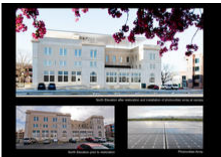
North Elevation - Photo Credit: Kevin G. Reeves (top photo)
