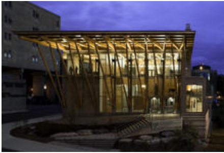
Main Entrance - Photo Credit: David Lamb Photography
