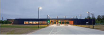
North Facade - Photo Credit: Frank Ooms
