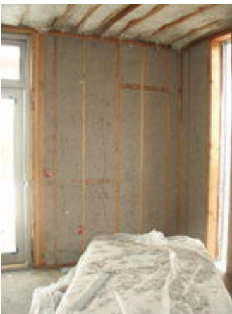
Finished install of the blown-in cellulose insulation - Photo Credit: Lawrence Scarpa
