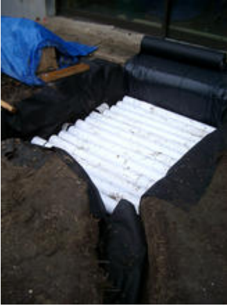
Installing the low tech stormwater system with stacked perforated pipe and gravel - Photo Credit: Brooks Scarpa
