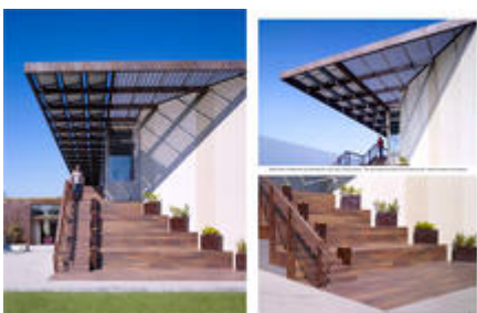
Amphitheatre steps leading up to green roofs and bedrooms - Photo Credit: John Linden
