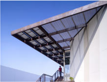
Detail of the large southwestern overhang with the 12kw solar system - Photo Credit: John Edward Linden
