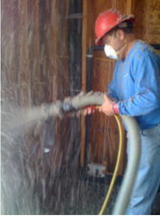
install of the 100% recycled blown-in cellulose insulation - Photo Credit: Lawrence Scarpa
