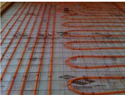
Thermally broken radiant slab ready for 50% flyash topping slab - Photo Credit: Lawrence Scarpa
