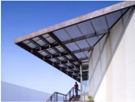
Detail of the large southwestern overhang with the 12kw solar system - Photo Credit: John Edward Linden
