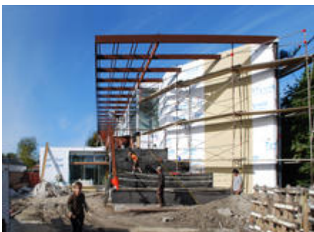
Construction view showing large overhang that shades the home - Photo Credit: Lawrence Scarpa
