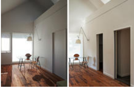
View of south window and winter light penetration (left). Conversely, the right images shows summer light penetration, as regulated by exterior shading device. - Photo Credit: Ken McCown
