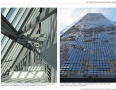
View of the uppermost floors of the northwest facade chamfered to allow sunlight to reach play area of elementary school to the northwest & view of Artist Ned Kah's "Firefly" installation that adorns the Wind Tower's north side. - Photo Credit: Photographs ©2012 Bruce Damonte. All rights reserved.
