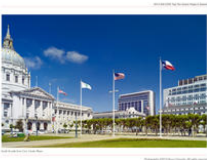
South facade from Civic Center Plaza - Photo Credit: Photographs ©2012 Bruce Damonte. All rights reserved.
