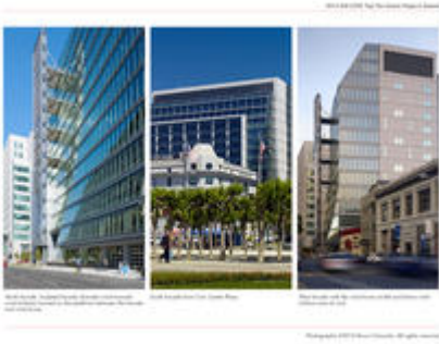
Exterior views of SFPUC - Photo Credit: Photographs ©2012 Bruce Damonte. All rights reserved.
