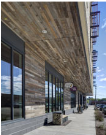
Overhang at South Facade -
