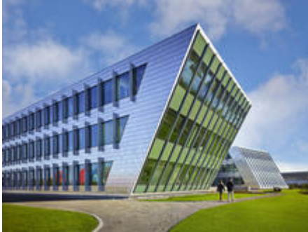
The orientation, tuned sunshade design, and massing optimize daylight while reducing solar heat gain. - Photo Credit: Benjamin Benschneider
